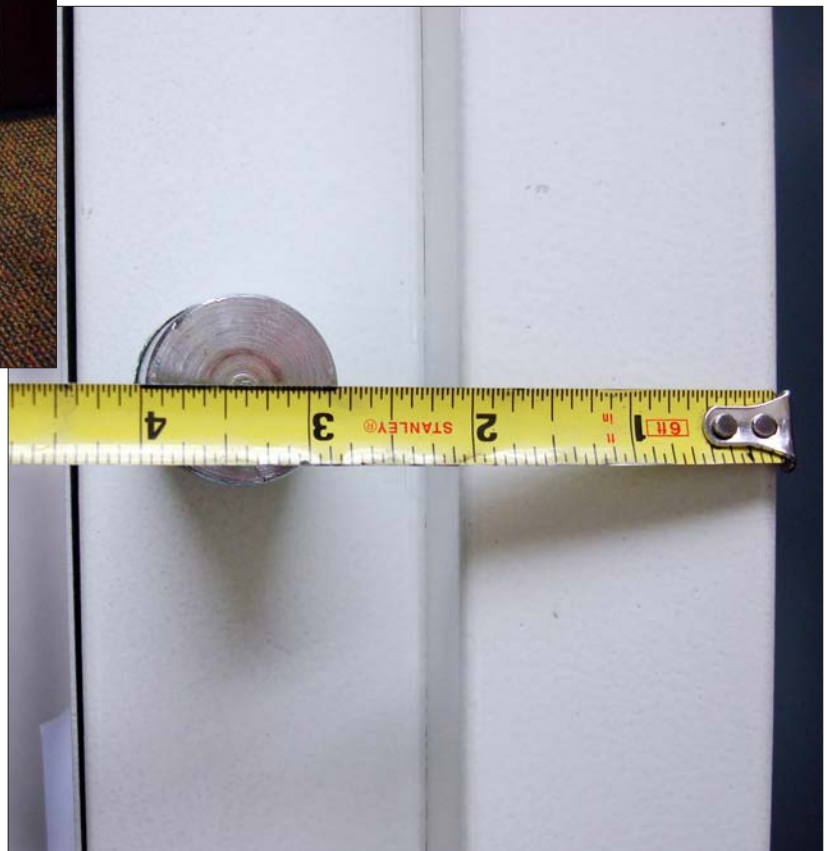
This is a useful photo to have for future reference. It tells us total door thickness as well as the depth from door face to the door bolts.
