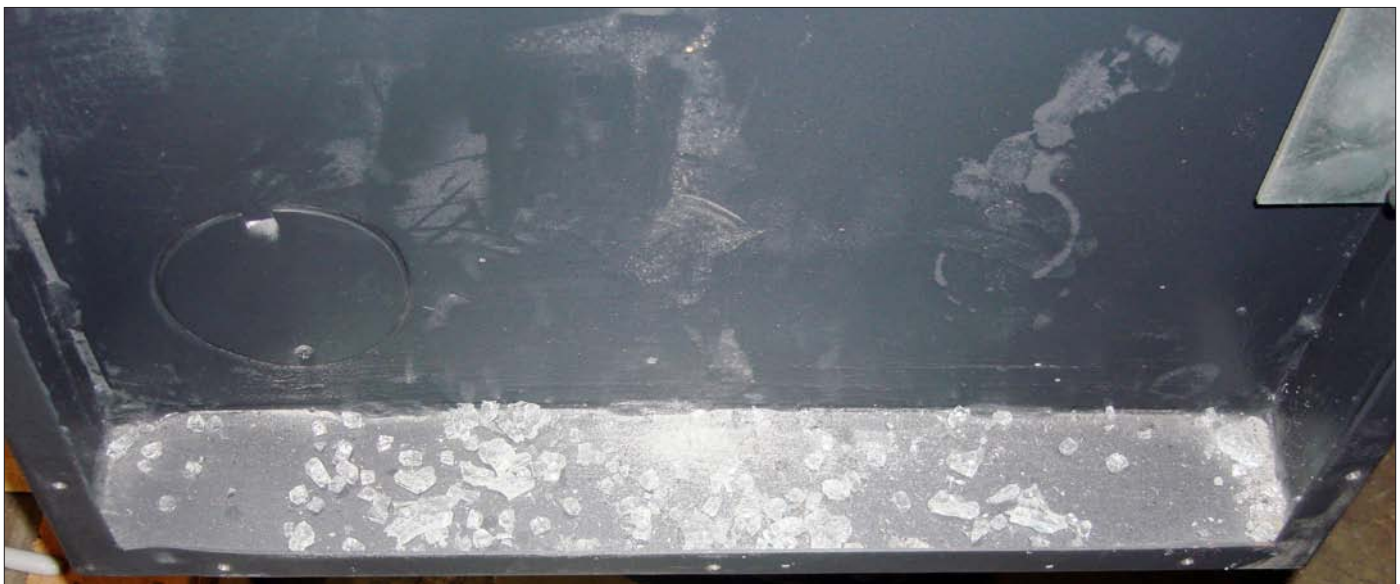
Glass in bottom of door.
