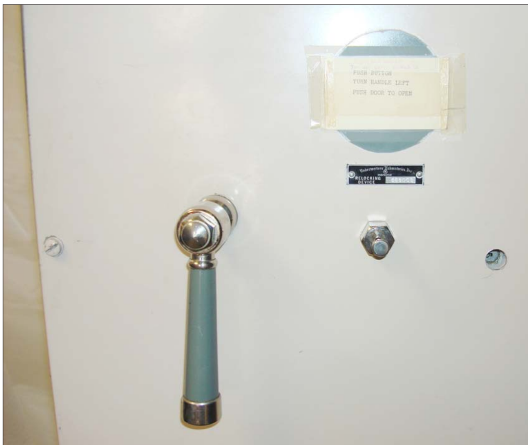
Emergency escape device on back of door.
