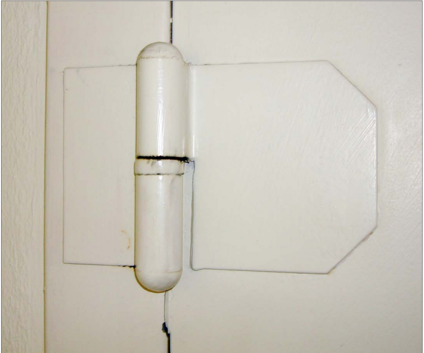
HHM hinge. Similar to the arrow-shaped straps used on some of their fire safes, but with the point squared off.
