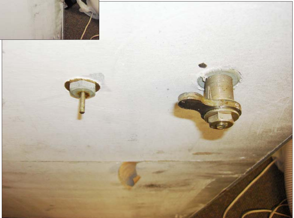
The plunger is on the left, the handle assembly on the right.
